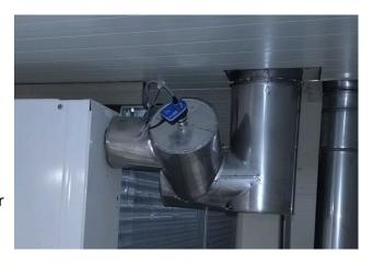
During the review at the cold store, a 44 kW evaporator designed to operate at -40°C with a circulation ratio of 3 was selected for detailed testing paired with our Vapor Quality Sensor. The evaporator's outlet pipe had a diameter of DN50, which was connected to a DN65 Vapor Quality Sensor. The piping configuration included a reduction back to DN50 and a riser pipe also sized at DN50.
