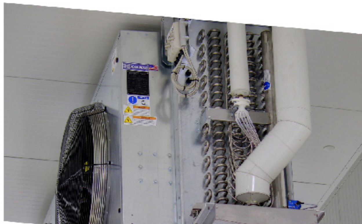
Vapor Quality installed on Air-cooled evaporator with distributor, Scantec Refrigeration
